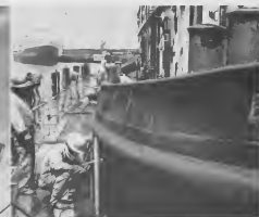
A LIFEBOAT from one of the tugs is swung away effortlessly, a toy for this crane, during the drydocking. Photo at right shows workers cleaning the upper section of the tug's hull as a tanker pulls into the gasoline docks in the background.
